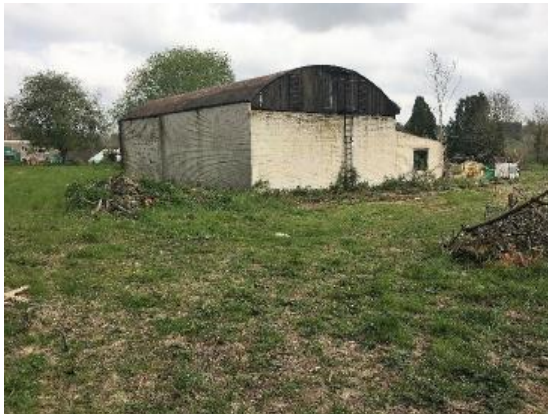
Dutch barn (Building 1)
