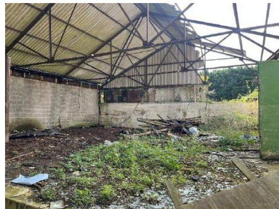
Former cold store building (Building 2)
